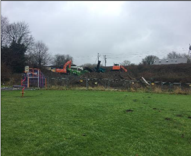
Photo 1: Restoration works in progress.
