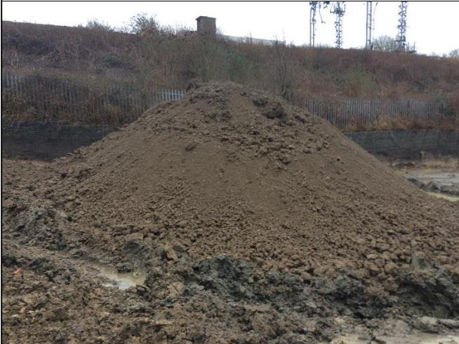
Photo 3. Clean imported top soil to be levelled over the site.
