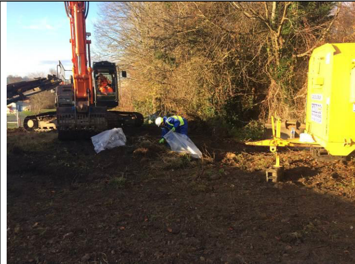
Photo 1: Hand picking of asbestos containing materials at surface.
