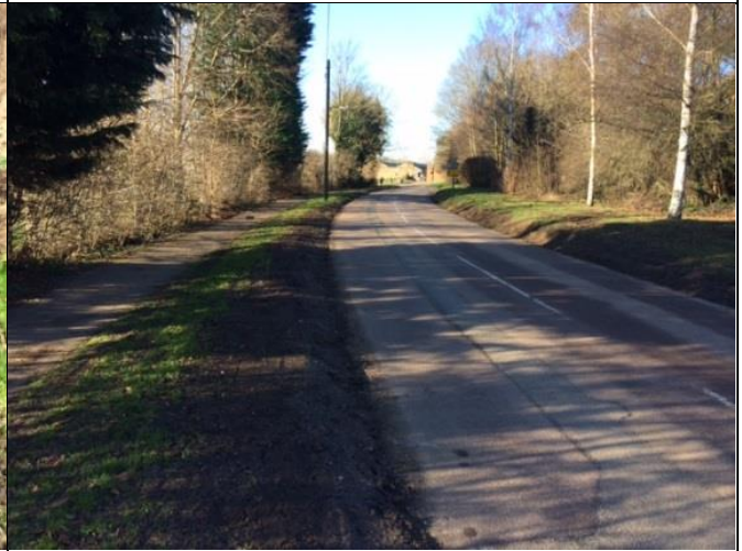
Photo 4. Repaired verges on Bridge Street.
