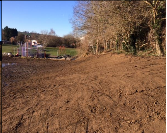
Photo 2. Photo of the completed slope leading down to the site.
