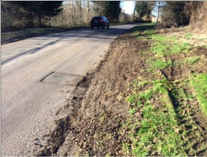
Photo 3. Repaired verges on Bridge Street.
